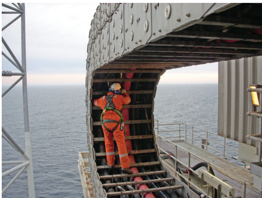
Inspection of hoses in Drag Chain performed by one of our service technicians.
